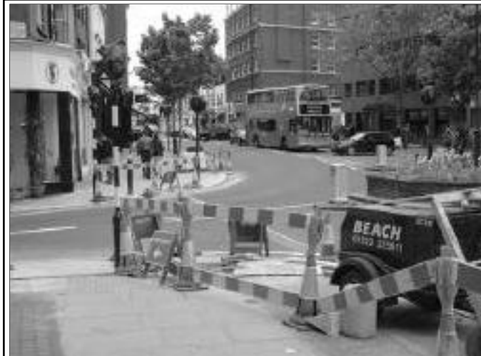
Work on the new crossing is in progress.
